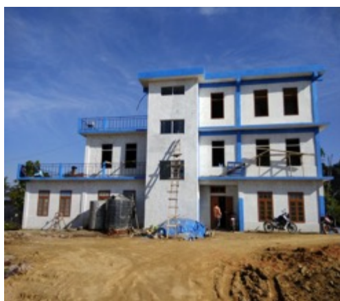
Photo22: Boys Hostel (Under Construction)
