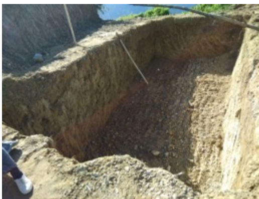
Photo24: Water Harvesting Structure (Under Construction)
