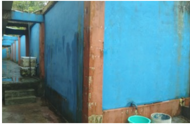
Photo19 : Water harvesting tank (Concrete)
