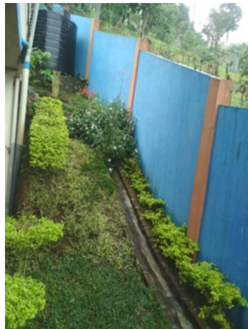
Photo16: Fencing with garland drain & Plantation
