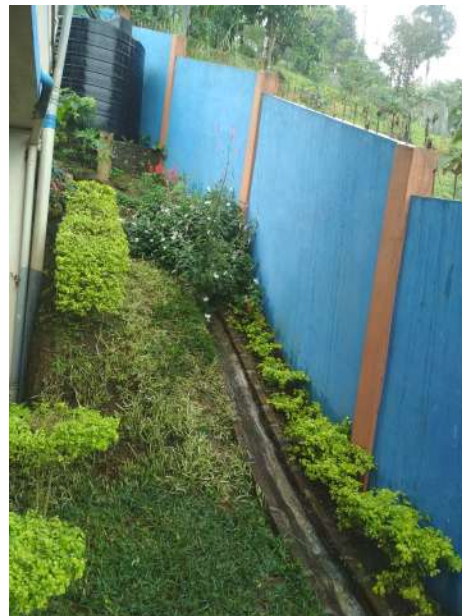
Photo16: Fencing with garland drain & Plantation
