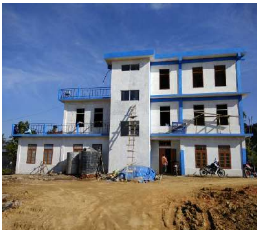
Photo 22 : Boys' Hostel (Under Construction)
