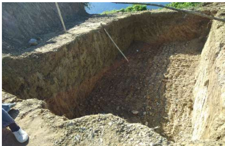
Photo24: Water Harvesting Structure (Under Construction)
